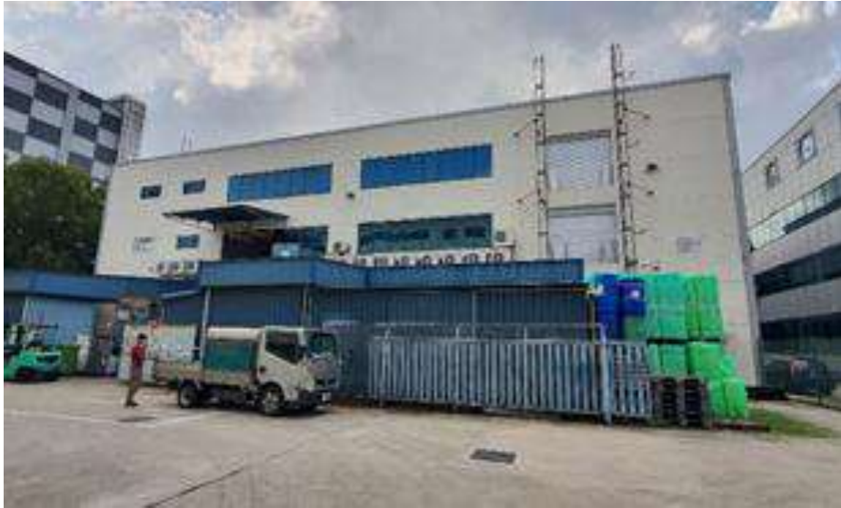
Existing property: 6 blocks of industrial facilities including warehouse, office and dormitory
